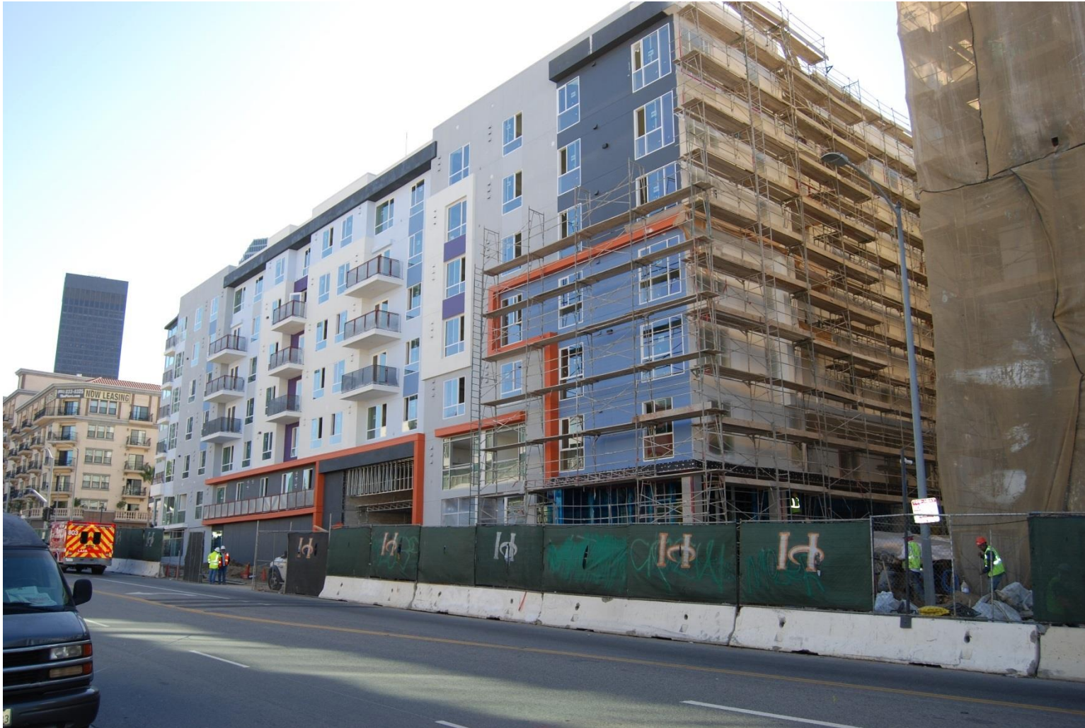
6. View of project site facing east on W. 6th Street.
