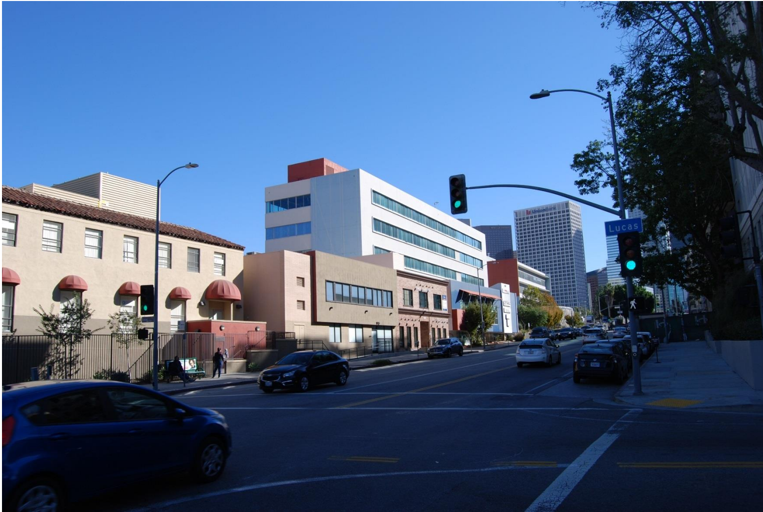
5. View of adjacent properties on W. 6 th Street northeasterly facing of the project site at the intersection of W. 6 th Street and Lucas Street.
