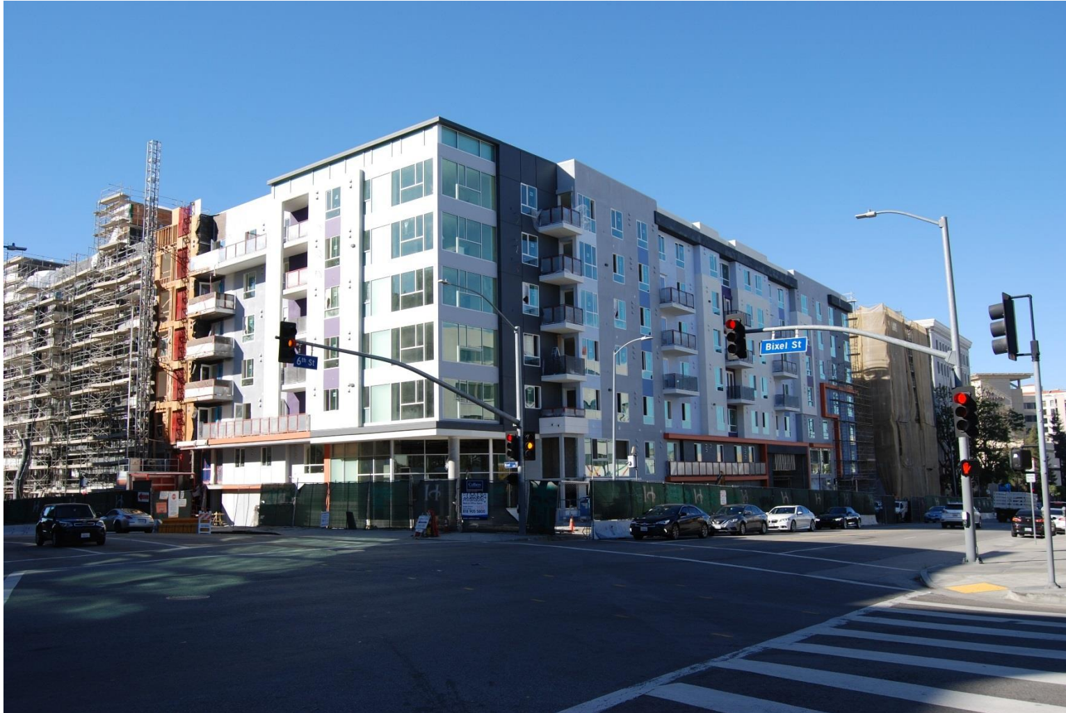
1. View of project site, southwesterly facing from the northeastern corner of W. 6 th Street and Bixel Street.
