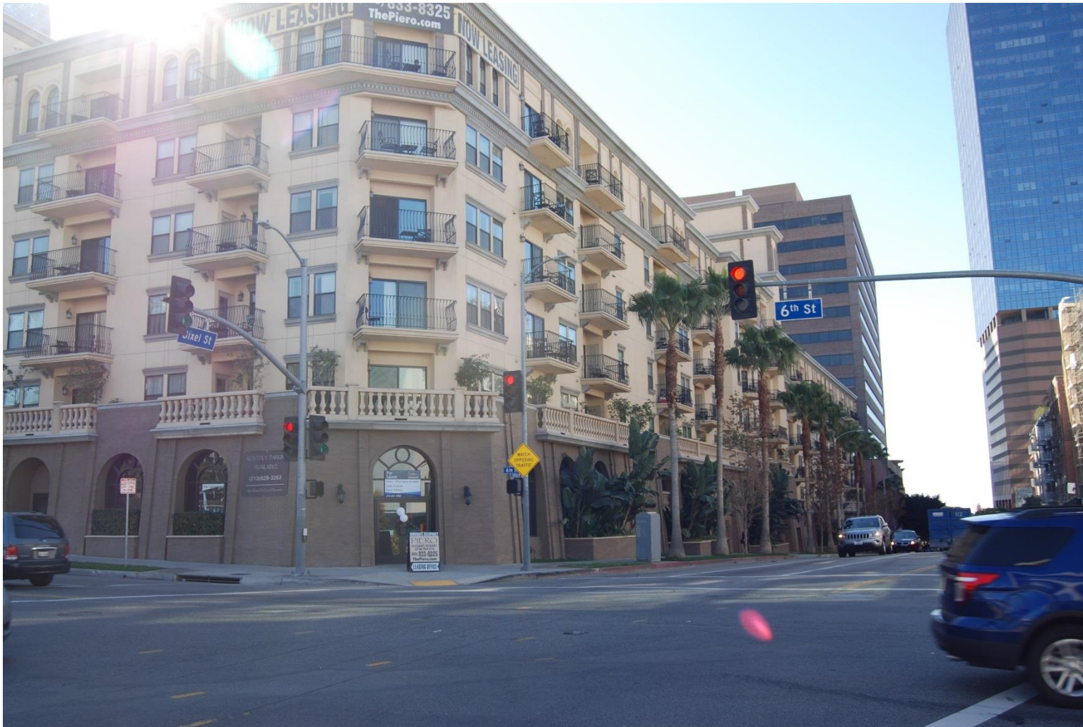
7. View of adjacent apartment building, southeasterly facing at the intersection of W. 6 th Street and Bixel Street.
